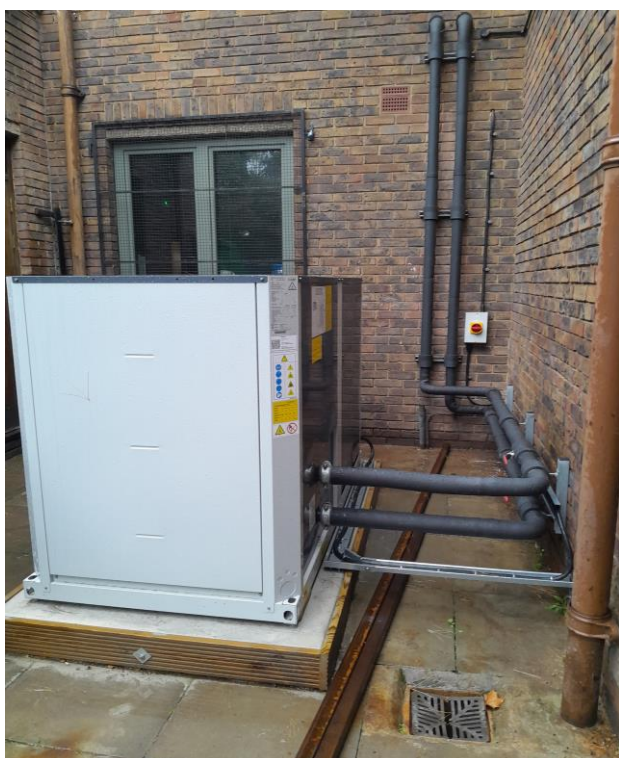
Air Source Heat Pump installation October 2023
